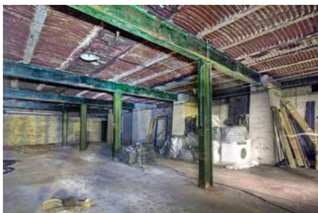
Steel propping is evident in the air-raid shelter
